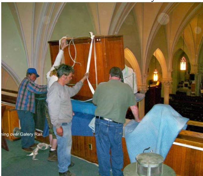
Moller console being hoisted from the main floor into the gallery
